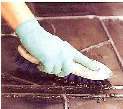
Cementing Process (Waterproofing)
