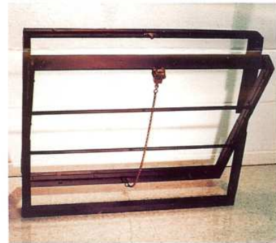
Overall view of frame after complete restoration.
